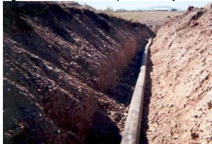
Figure 23: Trench Wall Sloped for Safety
