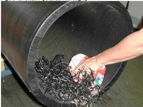
Figure 49: Clean Pipe Ends Thoroughly
