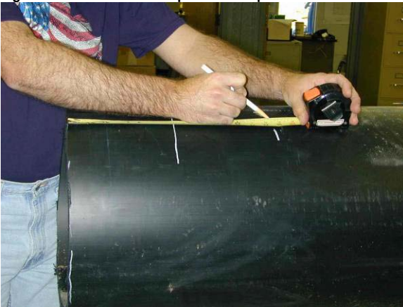
Figure 51: Mark Insertion Depth on the Pipe
