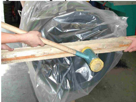
Figure 56: Installing Coupler on Pipe
