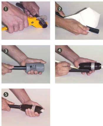
Figure 18 – Installation Instruction for Insert Type Mechanical Coupling
