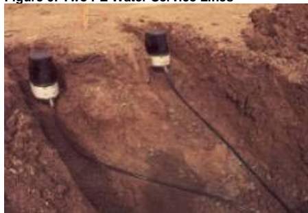
Figure 9: Two PE Water Service Lines
