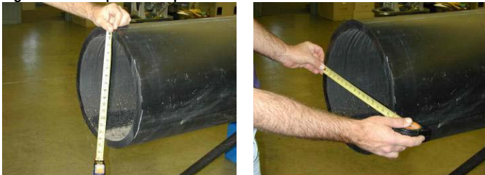
Figure 52: Cut Pipe Ends Square
