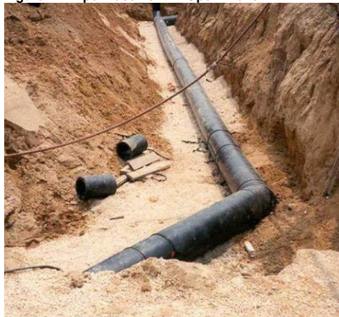
Figure 21: Pipe Placement in Open Trench
