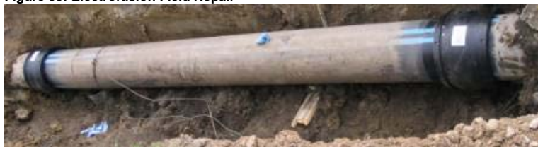
Figure 93: Electrofusion Field Repair
