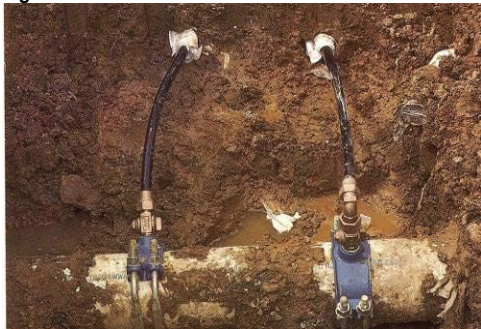
Figure 14: Mechanical Saddle Connection of PE Water Service Line to PVC Main
