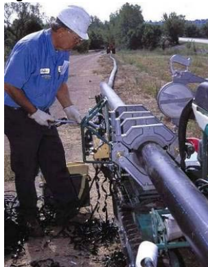
Figure 31: Butt Fusion of Water Pipe
