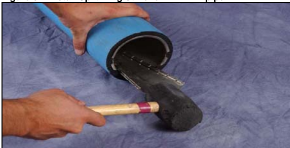
Figure 87: Install Split Ring Stiffener in HDPE pipe
