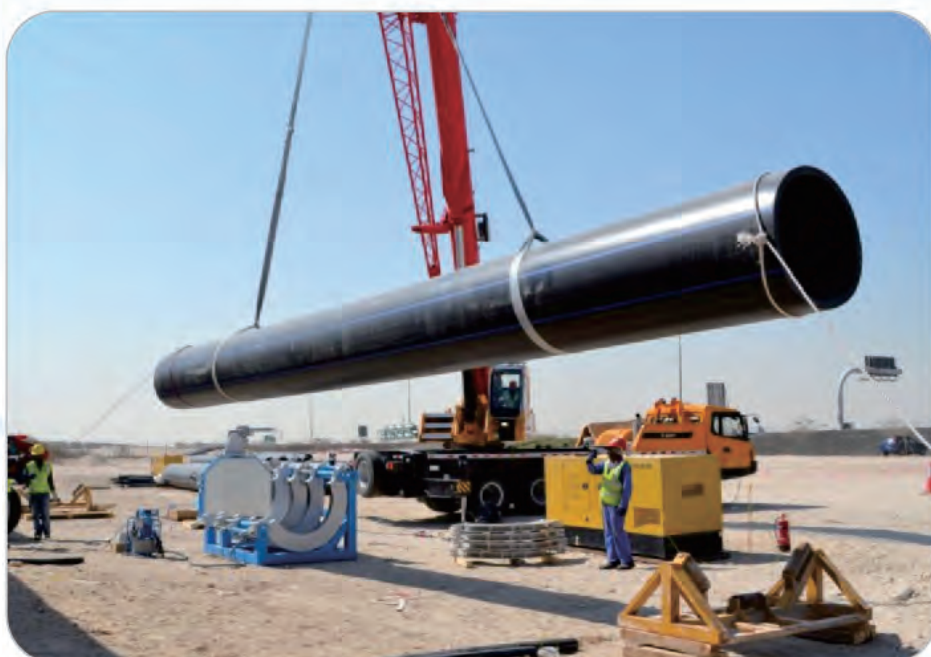
Petroleum Engineering: Corrosion-resistant piping system for UAE petrochemical plant DN1000, HDPE Pipe
